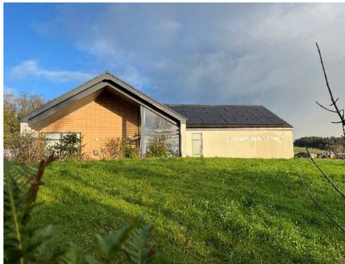
Figure 14: Community building installation of Solar PV and battery system.
