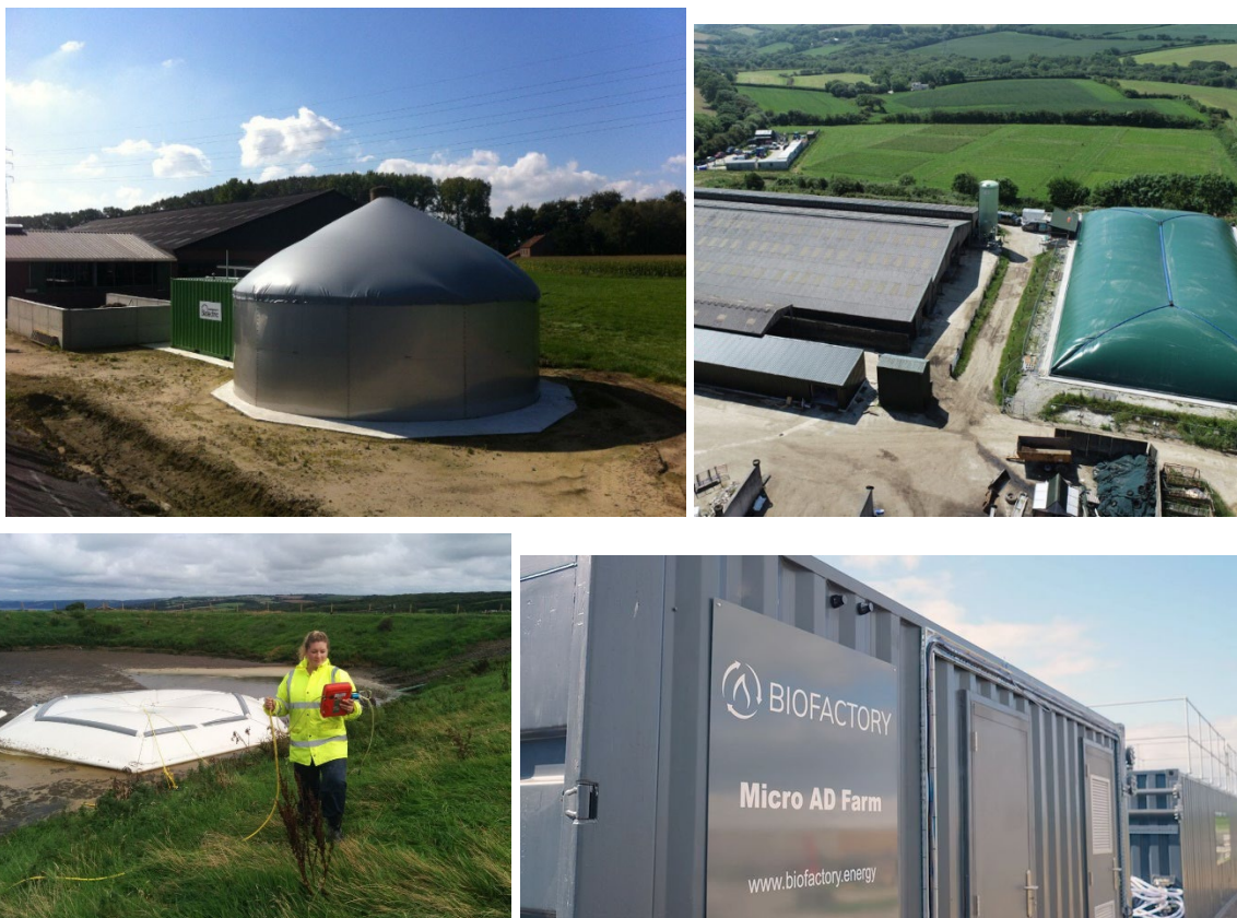
Figure 4: Micro-scale AD solutions targeting dairy slurry. From top left to bottom right: Dairy Energy (a micro-scale digester), Bennamann (a covered slurry lagoon), Qube (a partially-covered lagoon) and Biofactory (a containerised digester).
