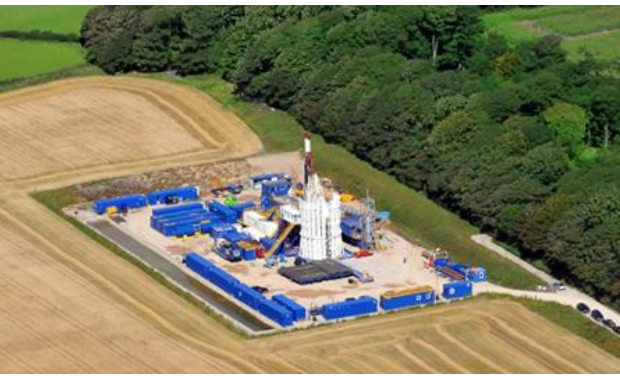
1. Drilling & fracturing few weeks/well - largest footprint
