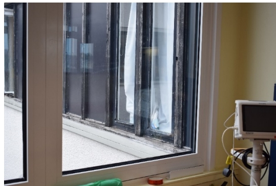
New double glazing in corridors (only non-openable units replaced)
