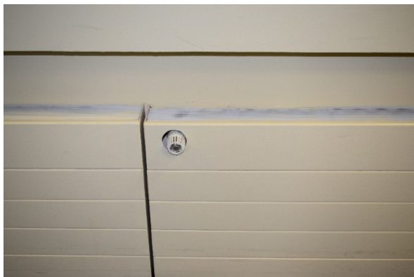
Radiator Type 1 - Low surface temperature (LST) in a corridor (not typical in the hospital)
