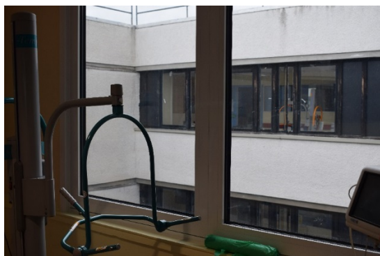
New double glazing in corridors (only non-openable units replaced)
