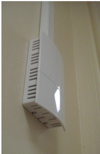
Wall mounted heating zone control temperate sensor (1 of 2) in east corridor
