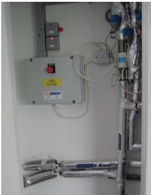
Image showing the emergency 'isolation' push-button and associated controls and services supplying an individual single room. Each room has this function and the control are located within a services cupboard (accessed from the corridor) adjacent to each single room
