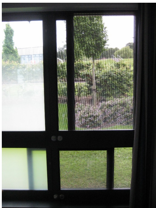
Example of the 'new' style (post-retrofit) window with independent and variable opening, top and bottom, side-sliding sections complete with security mesh
