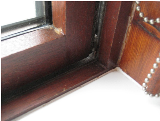
Examples of poor fitting windows (LHS) and faulty catch (RHS)
