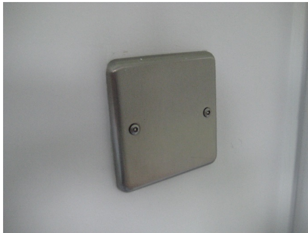
Image showing the metal fascia plate behind which sits a thermistor which acts as the room heating control thermostat
