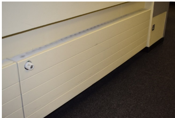
Radiator Type 1 - Low surface temperature (LST) in a corridor (not typical in the hospital)
