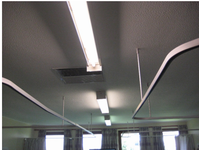
Tilt and turn window within a south elevation single room (LHS). Ceiling and bank of 4 x windows within a north elevation 4 bed room (RHS) – this also shows the supply air ventilation grille and light fittings.
