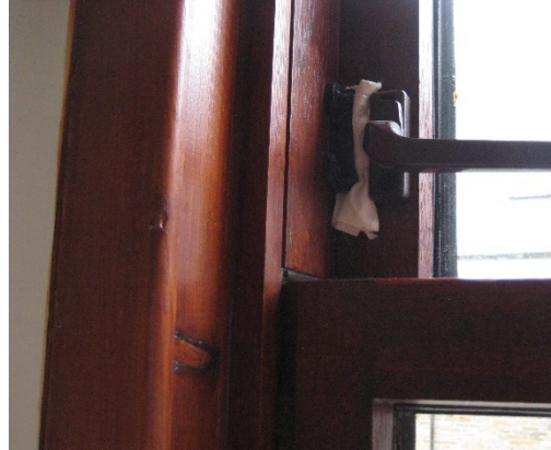
Examples of poor fitting windows (LHS) and faulty catch (RHS)
