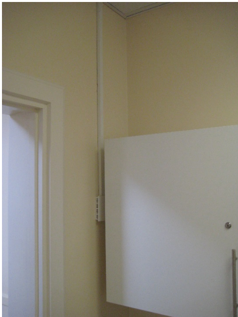
The heating control temperature sensor (2 of 2) in the west corridor with the carbinet installed directly inadjacent.
