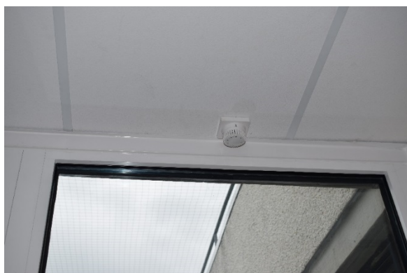
Radiant panel thermostatic control in ceiling
