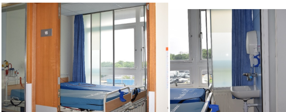
Single room (without ensuite (sink only) – showing secondary glazing and curtains
