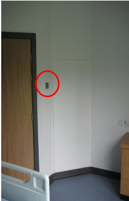
Image showing the metal fascia plate behind which sits a thermistor which acts as the room heating control thermostat
