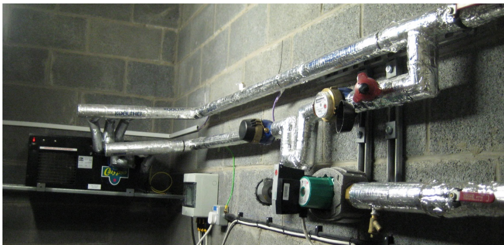
Example of an 'in-line' chiller (the black unit on the LHS of the image) installed on the mains cold water supply to a ward unit.
