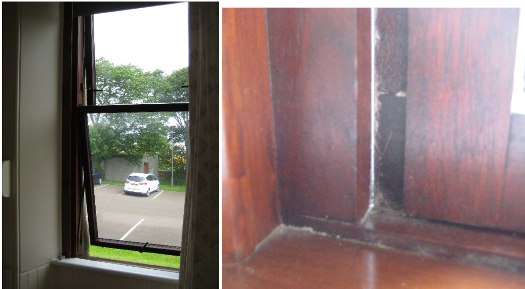
Windows openable at bottom section and/or top (LHS). Poor seal evident when in closed position (RHS)
