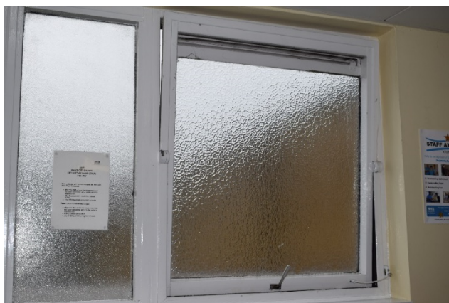
Openable (100 mm) window in a corridor fitted with restrictor
