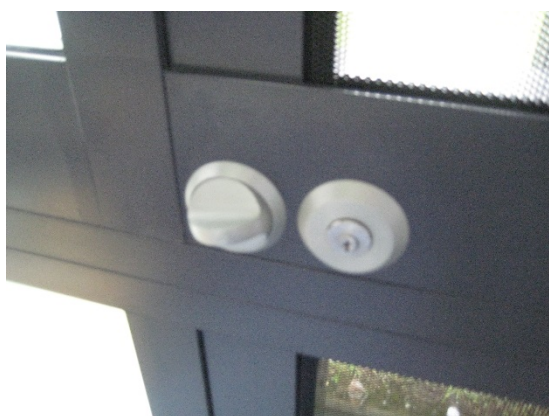
Thumb-turn control of the side-slide opening sections and associated lock
