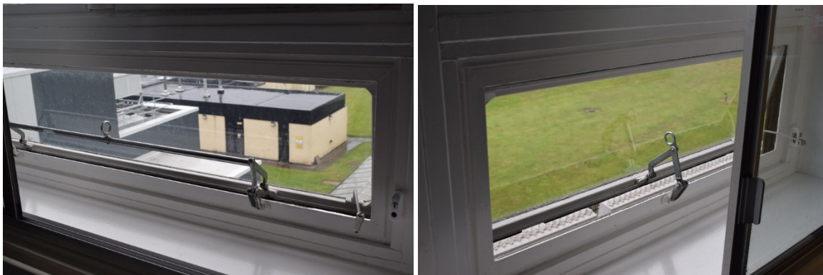
Openable lower section – although sometime ‘stuck’ either fully opened or closed.
