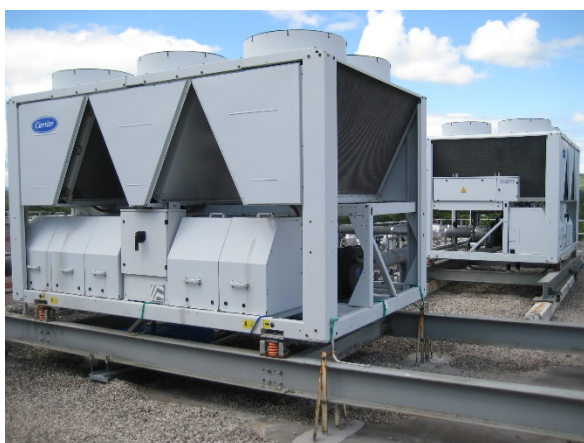
Roof mounted chiller units (which include some spare capacity) (RHS)
