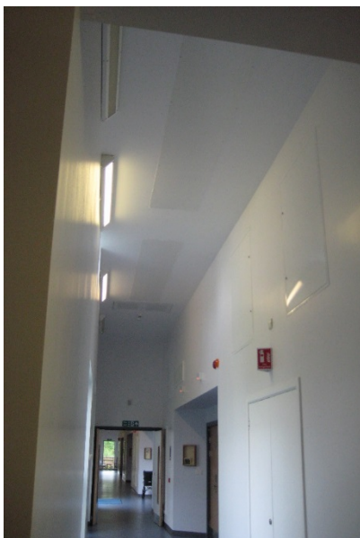
A typical corridor with high level, ceiling mounted radiant panels, with access to the single rooms
