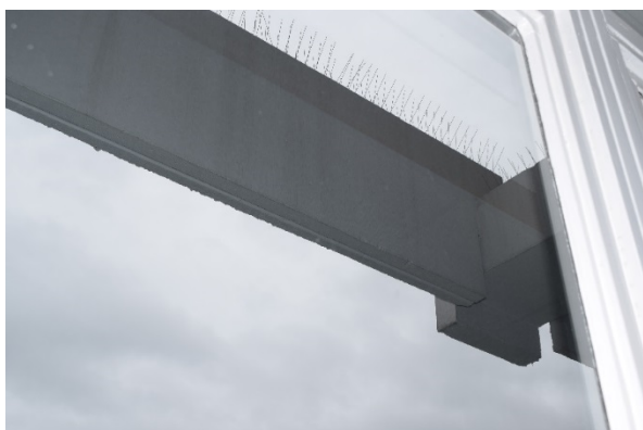
Concrete external shading
