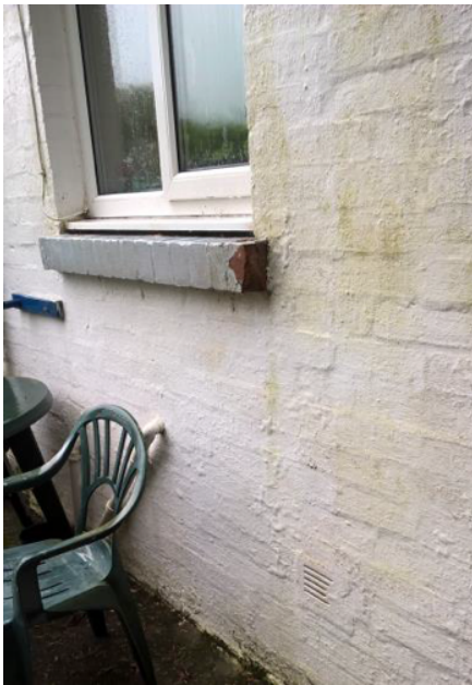
Photo 3: Extension wall construction showing thickness of wall. Condensation is visible on inside of kitchen window.
