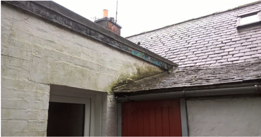
Photo 2: Flat roof to extension, join of pitched roof to extension (kitchen door)
