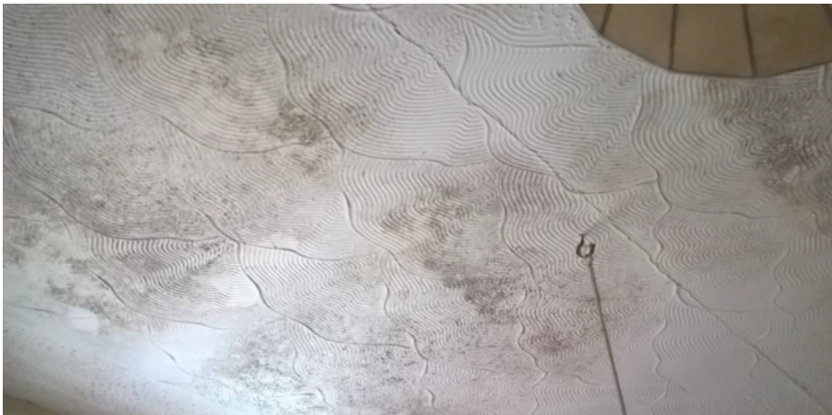
Photo 1: Mould on kitchen ceiling under flat roof
