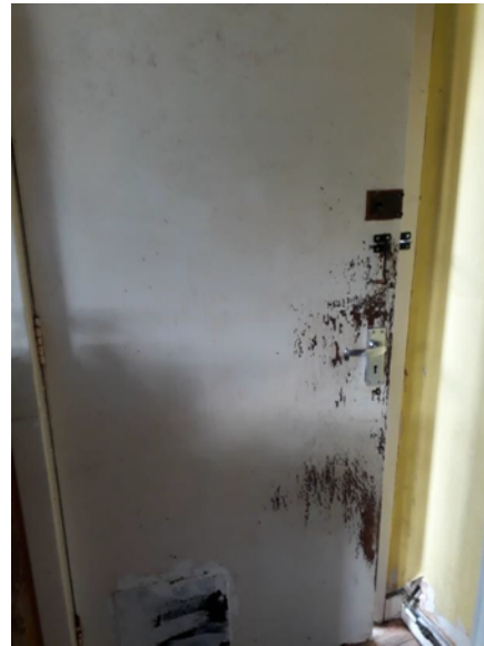
Photo 2: interior door used for exterior door
