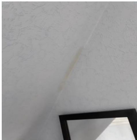
Photo 4: Damp on upstairs bedroom ceiling
