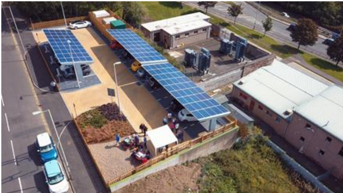
Figure 2: Integrated solar, storage and charging hub. Dundee, Scotland. Sourced from Drive Dundee Electric (2019).
