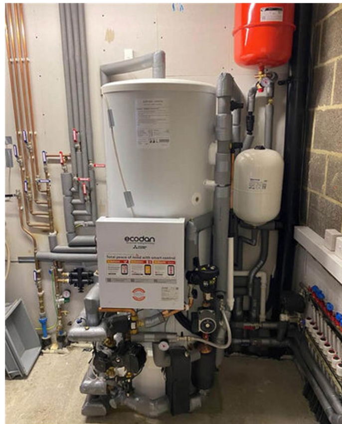
Figure 2: In-situ thermal store 31
